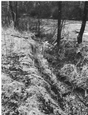
Airport Stormwater Discharge to Spring Creek
